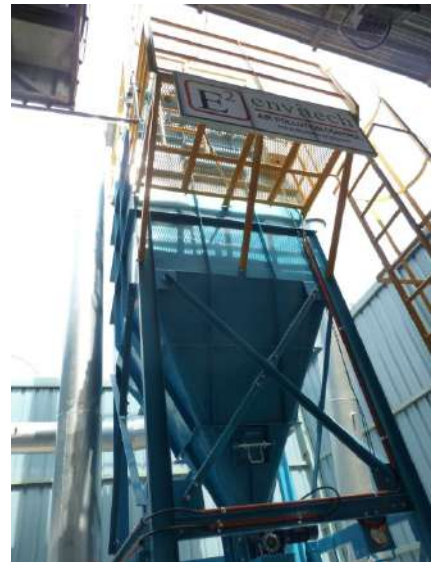
4000 cfm Jetpulse Dust Collector
