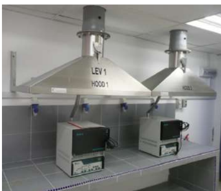
Stack Inspection & Monitoring
