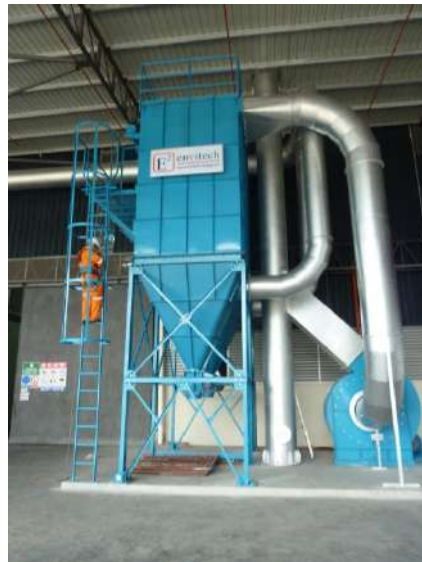
17400 cfm Jetpulse Dust Collector
