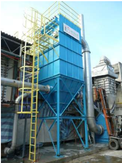
12000 cfm Jetpulse Dust Collector
