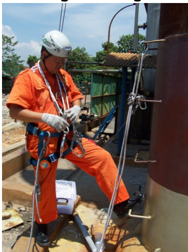
Left: Scaling and inspecting 40m ht chimney for battery recycling plant
